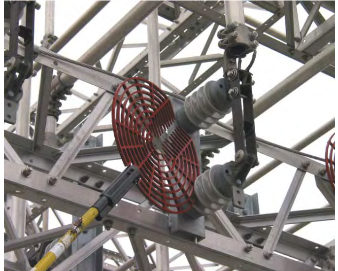
Figure 9: Install with Smooth & Steady Push
