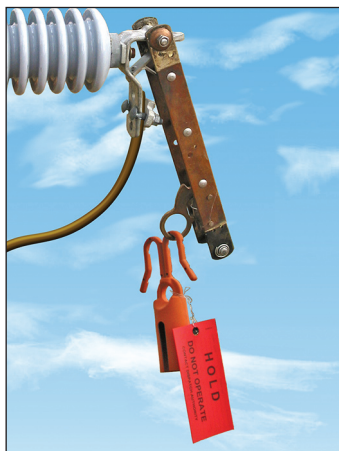
R-TD installed on a disconnect switch
