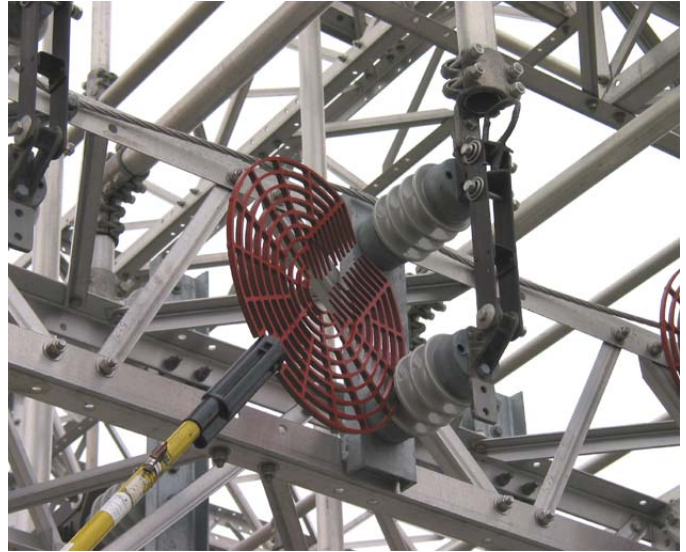
Figure 9: Install with Smooth & Steady Push
