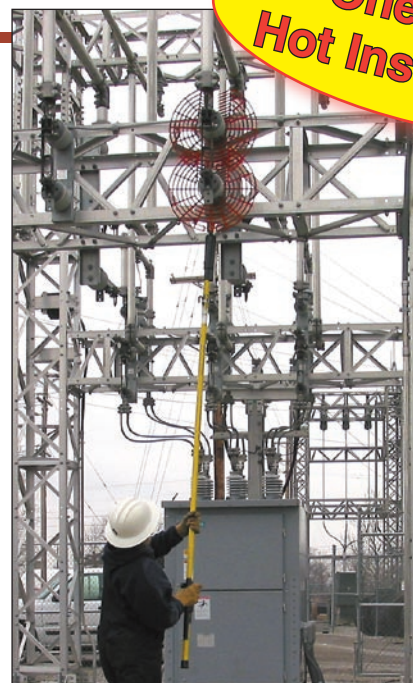
Model W-002R Being Installed in a Substation
