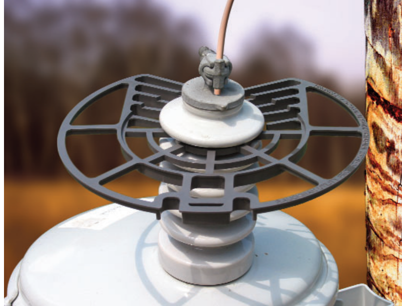
Model W-1525G ZAPshield Installed on a Distribution Transformer.
